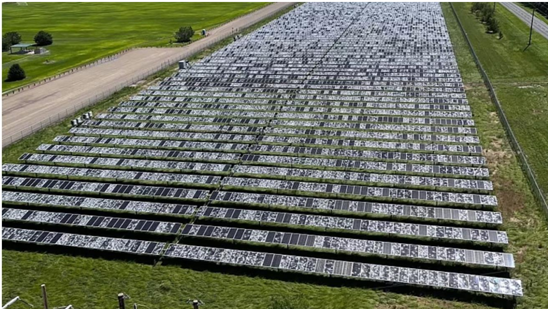
Baseball-sized hail hit this Scottsbluff solar farm Monday at 100 to 150 mph. (Courtesy Photo)
